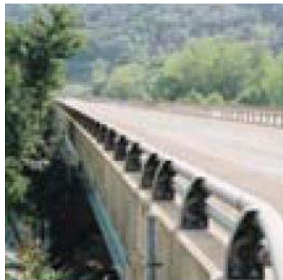
Athens Bridge - Pennsylvania.
