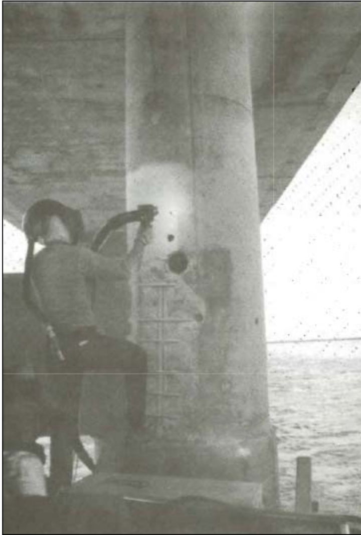
Niles Channel Bridge
